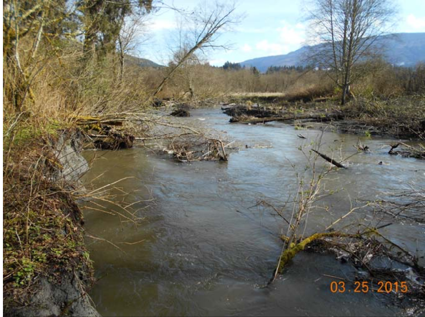
Photo 1 - View north showing active channel and cut left bank. Note erosion and recruitment of woody debris into channel.
